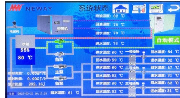
Air compressor waste heat recovery system
